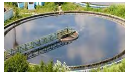
Municipal and Industrial water & wastewater treatment
