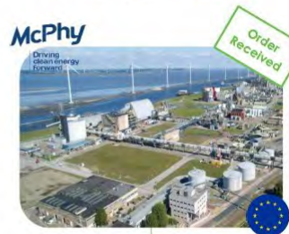
Delfzijl Industrial Park – The Netherlands
