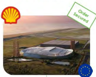
Hydrogen Holland I Project (Largest Hydrogen Project in Europe)
